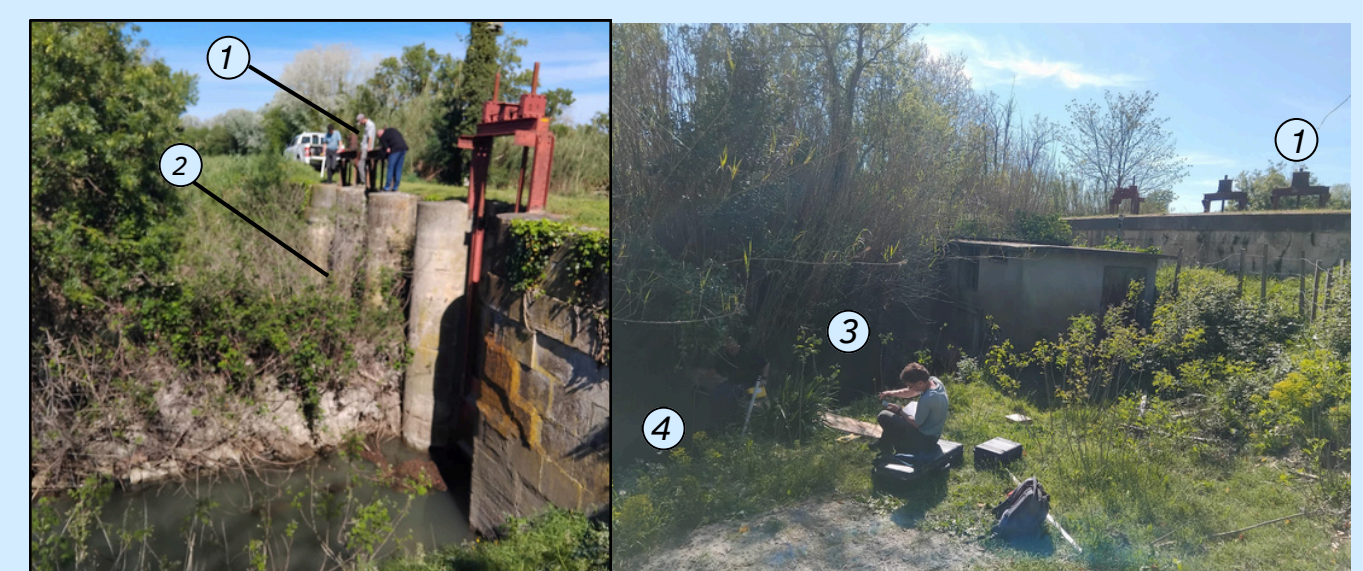
Control flow sluice gate (1) Upstream pslb Dragino pressure sensor (2)
